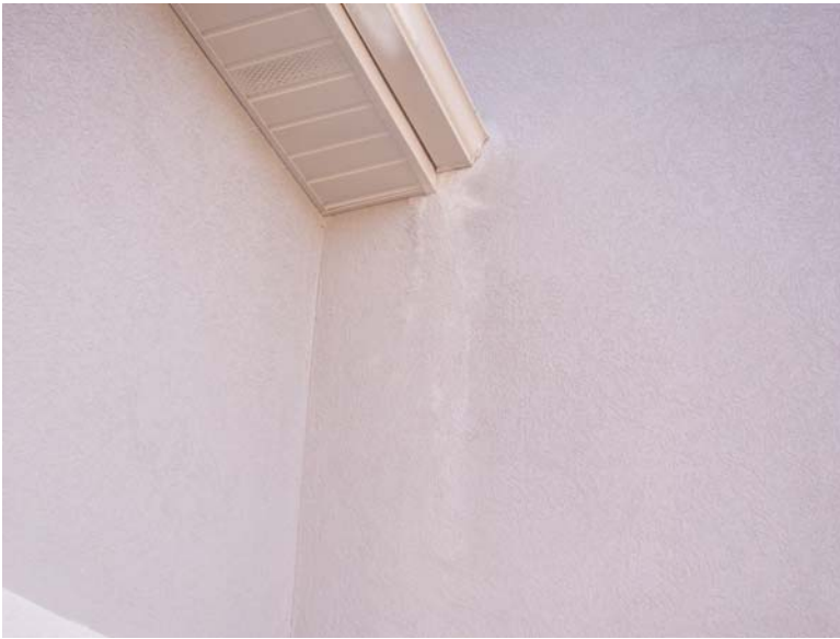
silicone around gutter to help keep water from washing down stucco
